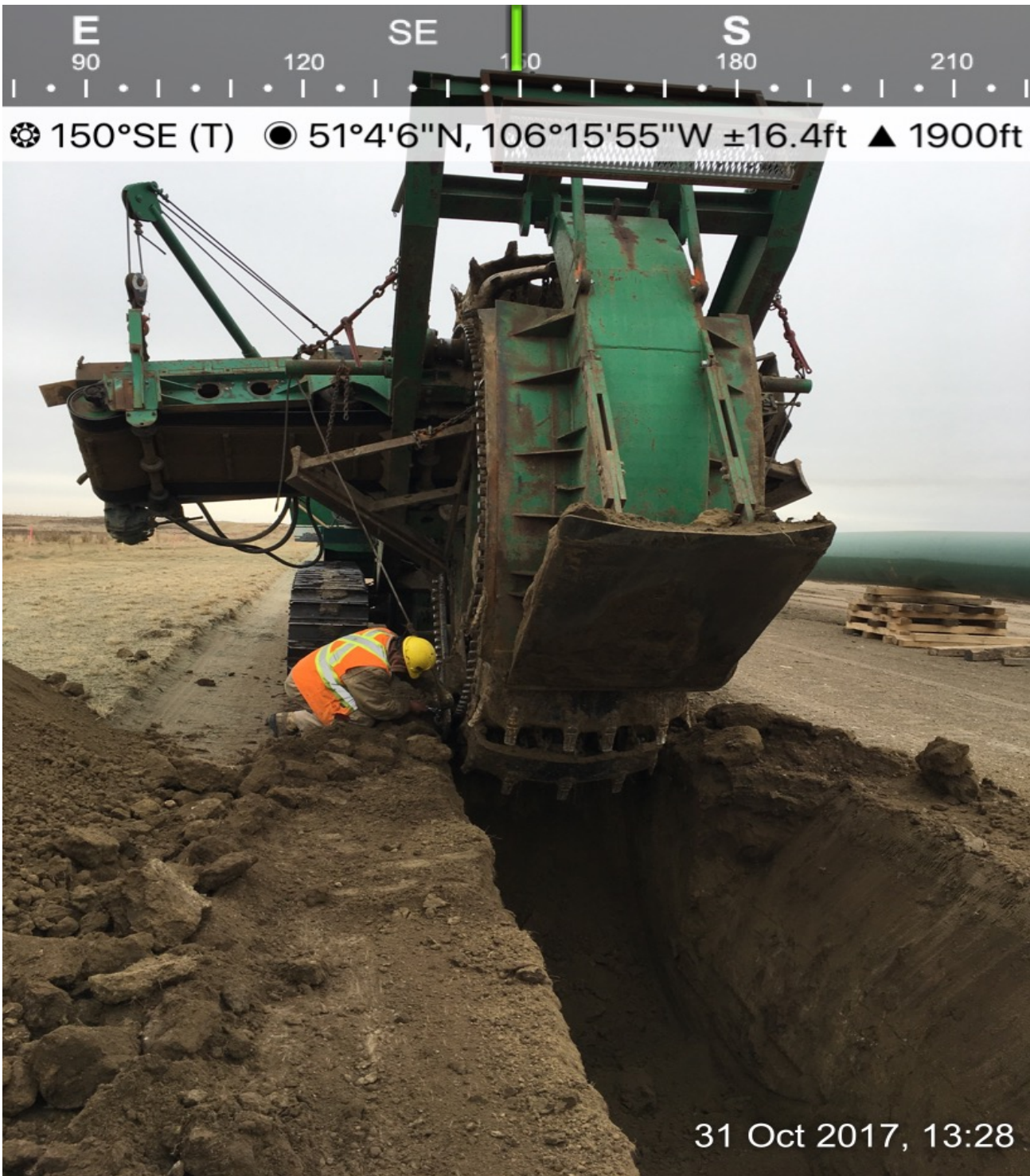
DITCHING MACHINE AT KNOWN TRADITIONAL AREA
