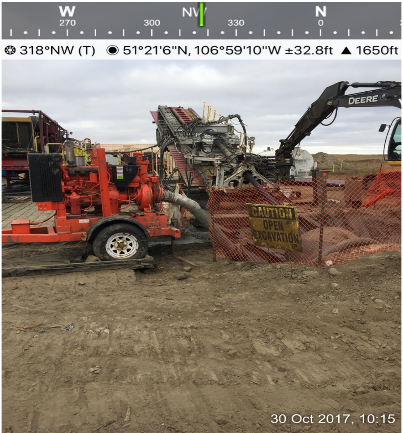
HORIZONTAL DIRECTIONAL DRILLING AT SOUTH SASKATCHEWAN RIVER
