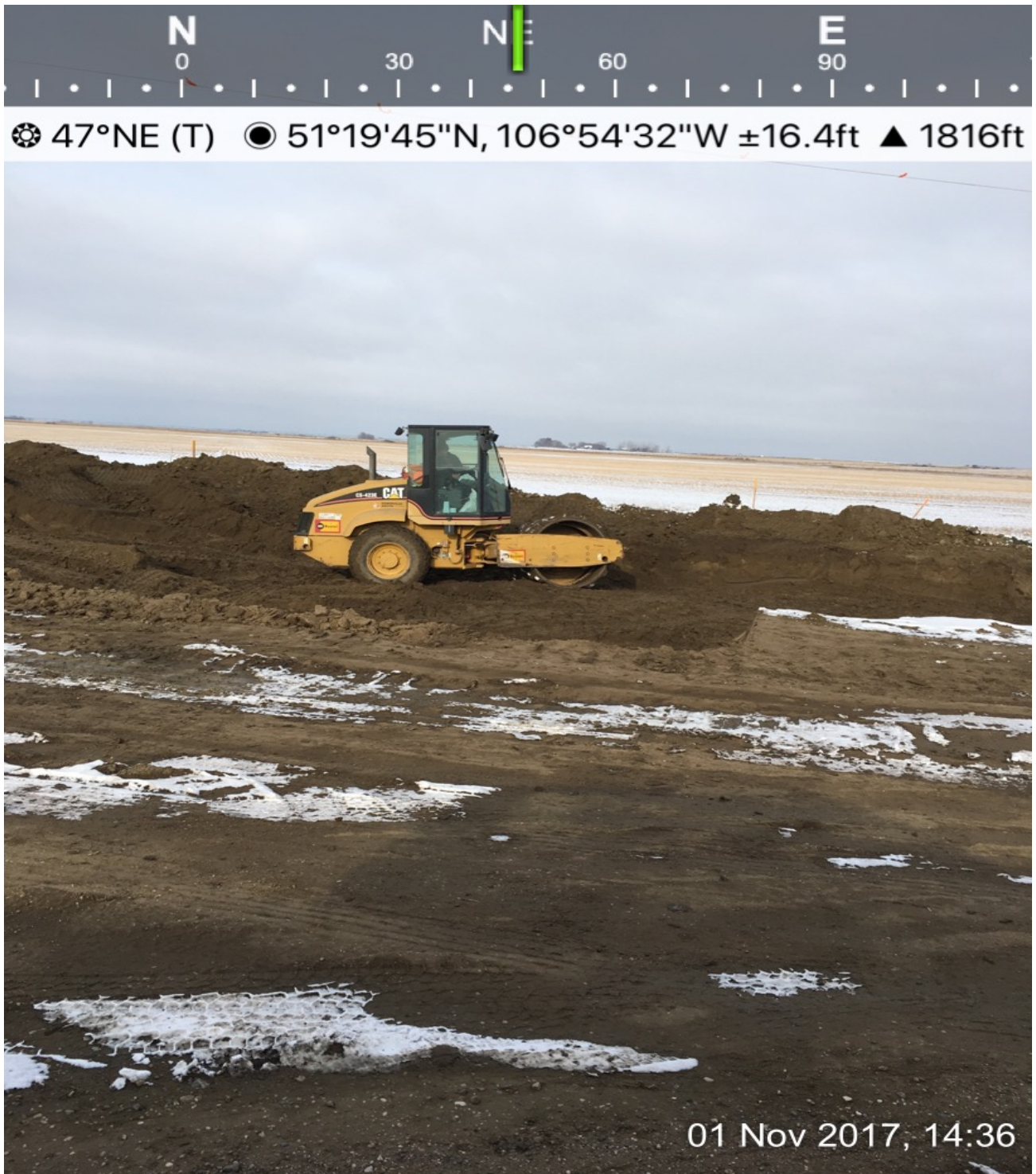
COMPACTION OF SOIL
