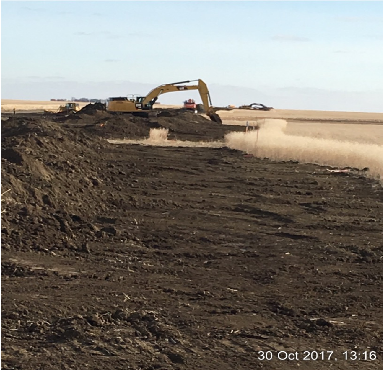
PULLING TOPSOIL BACK ONTO THE RIGHT OF WAY
